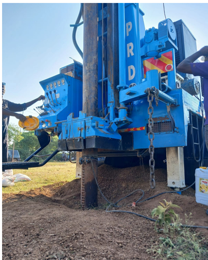
Installation of surface casing at Sango Primary School
