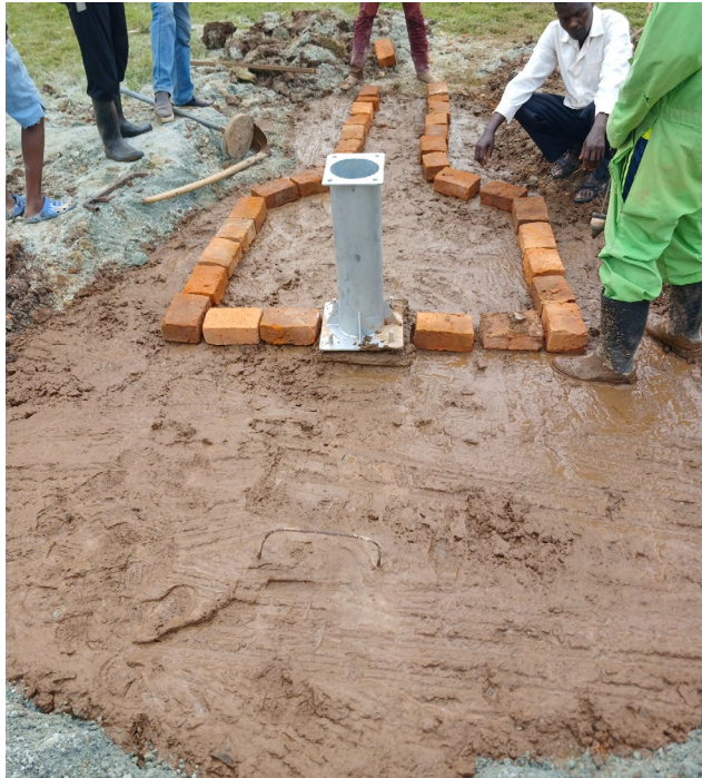
Ongoing Pad Construction
